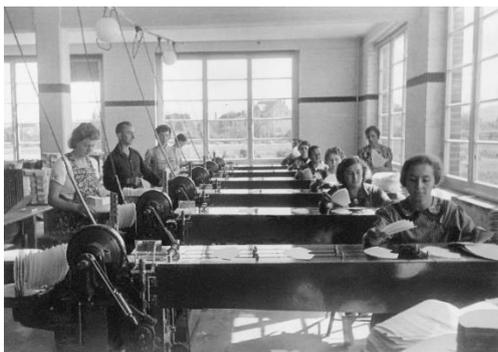
Image 4: In the early days of coffee filter production women folded the filters with the help of templates, the rest was done by the punching machine.
