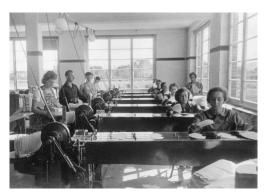
Image 4: In the early days of coffee filter production women folded the filters with the help of templates, the rest was done by the punching machine.
